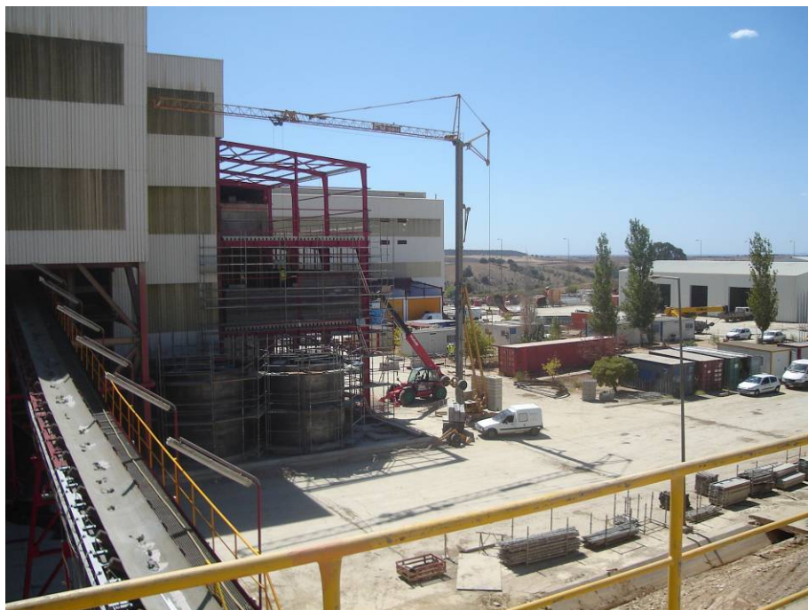
Figure 18.2: General View of Aljustrel Concentrator being Refurbished.
