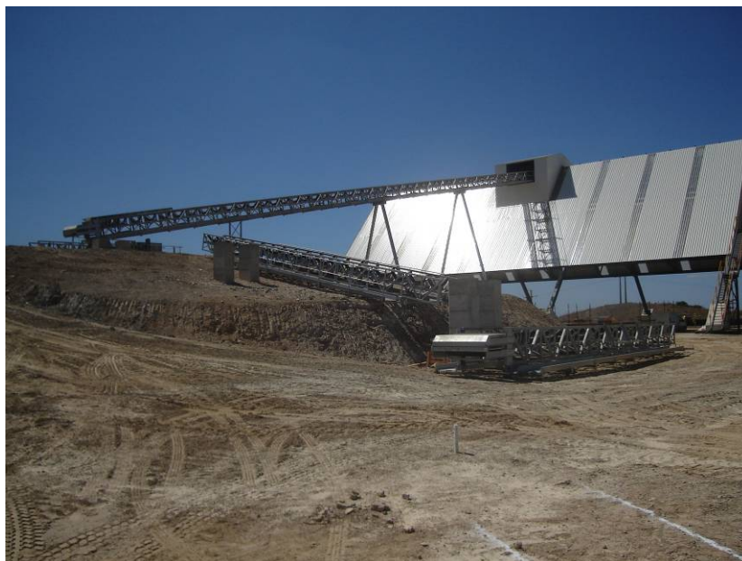
Figure 18.1: Covered Crushed Ore Stockpile under Construction
